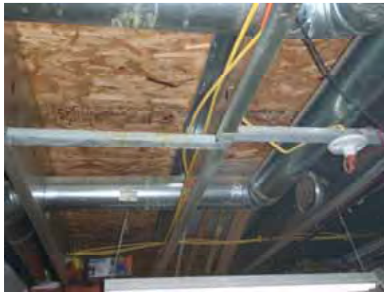
Residential use of cold form steel with penetrations and 24" on center
