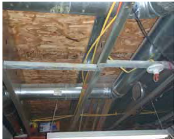
Residential use of cold form steel with penetrations and 24" on center
